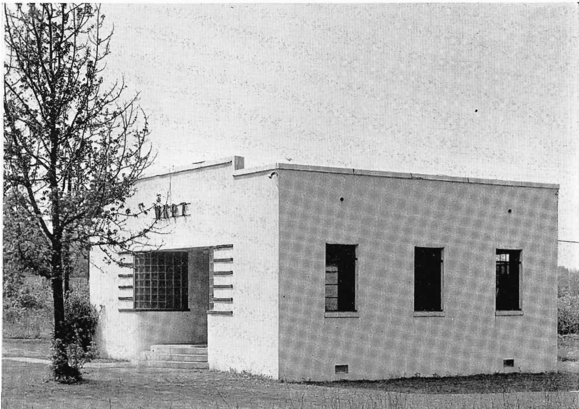
FIG. 7. The WKPT stuccoed tile transmitter building is located 2½ miles from Kingsport.
