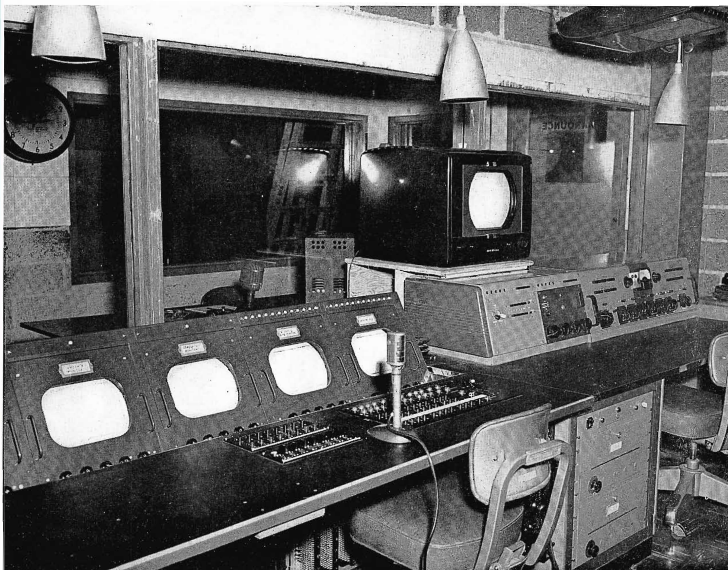
FIG. 15 (below). View of Control Room "C" showing arrangement of technical equipment. Program Director's Console with switching facilities is at left and Audio Console at right.
