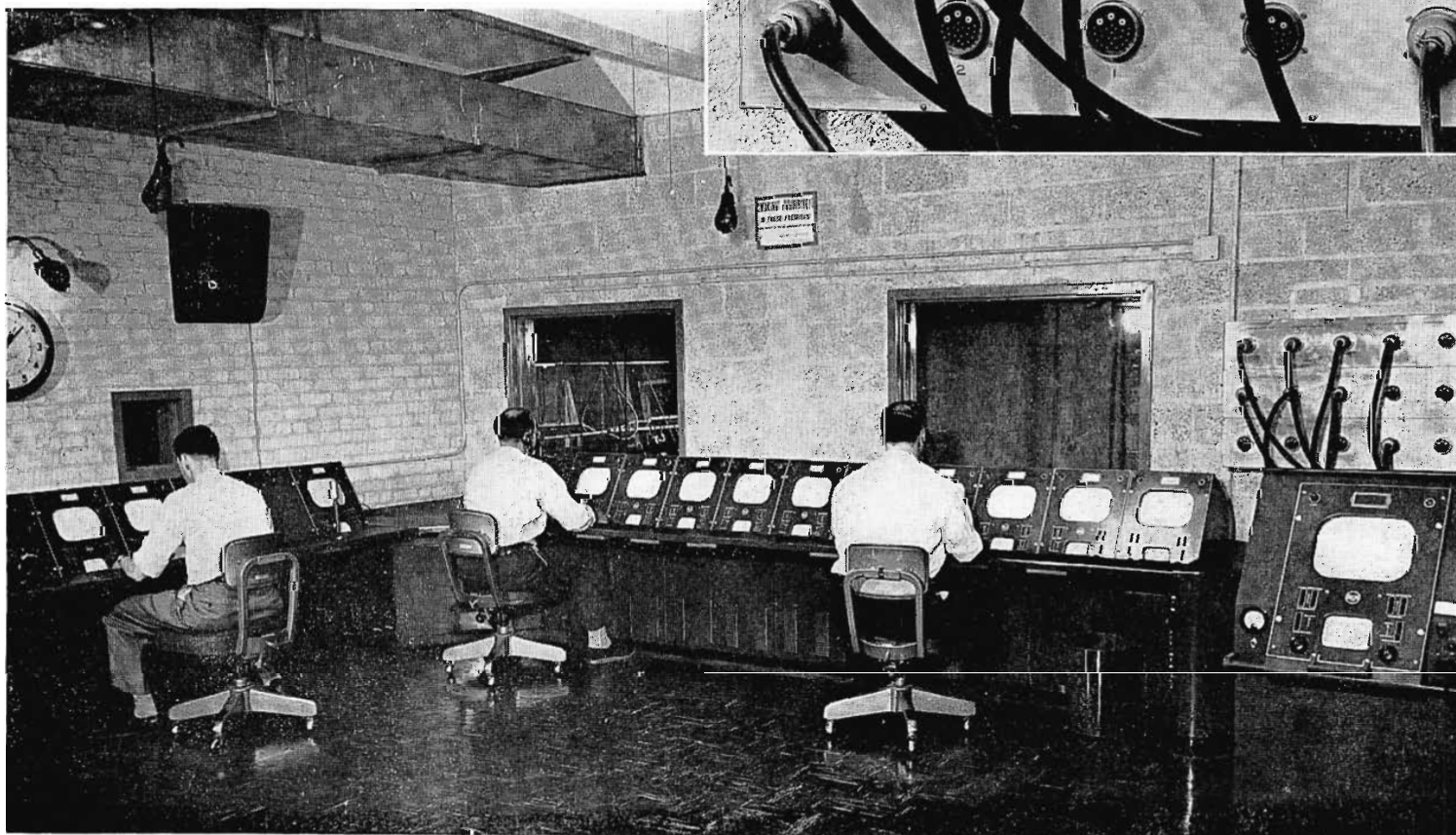
FIG. 29. The studio camera shading and monitor controls are centrally located in this console. At the extreme left part of the film shading and monitor controls are also visible.
