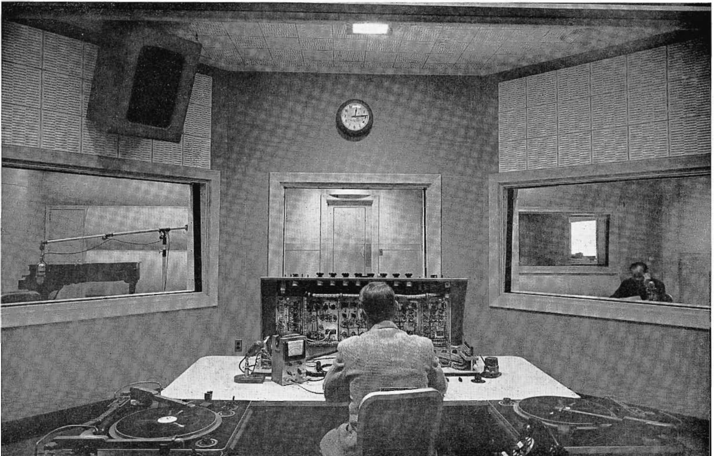
Large windows in the control room shown below provide good visibility into all three studios. This photo was taken from the transmitter room. ▶
