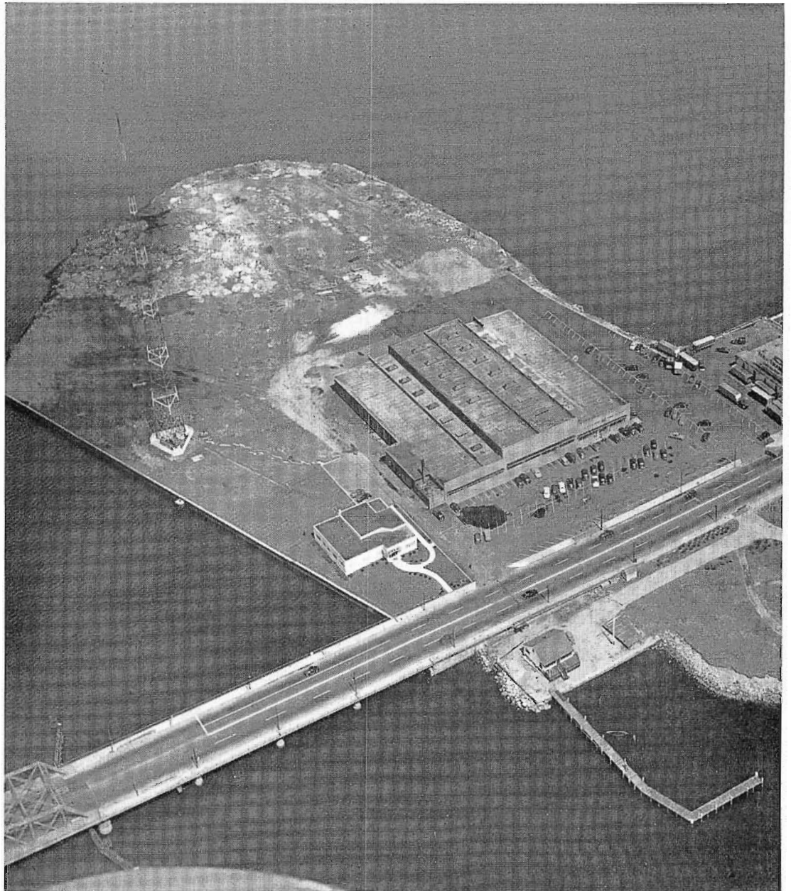
Air view of Pope's Island and part of New Bedford. The WBSM transmitter building and antenna (left center) are entirely surrounded by the salt water of Buzzards Bay.
