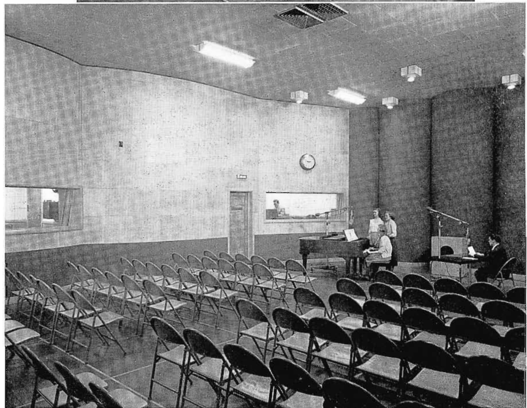
FIG. 4 (at right). Studio "A"—looking into Sub Control room and Master Control room.
