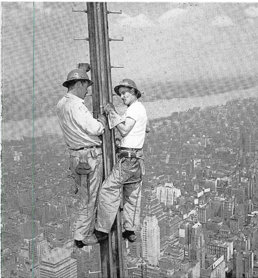
3 Before dismantling of the old TV antenna began, temporary antennas were erected to insure continuous service. Pat Corbet (right), 57, and son, Joe, 32 years old, are fastening transmission line on NBC's temporary antenna.
